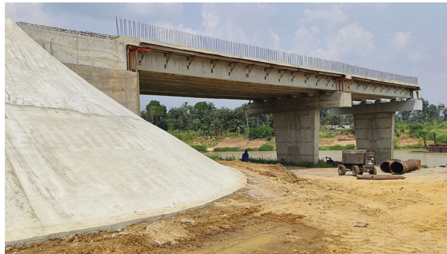
POLAKU-SABAGREIA ROAD, BRIDGE ONGOING
