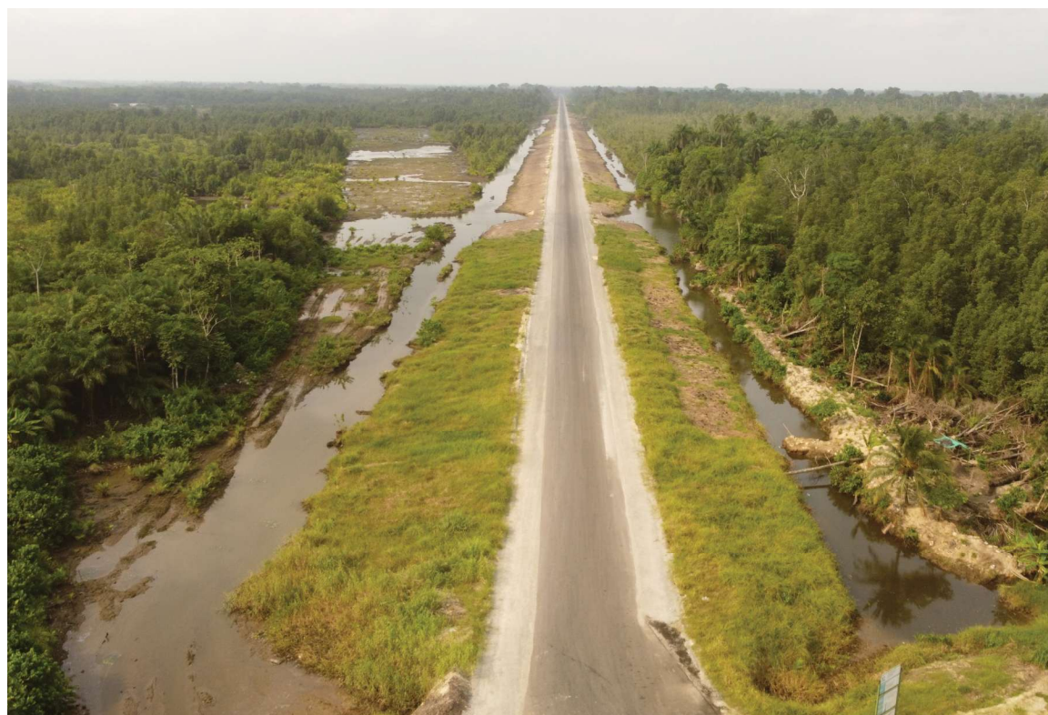
NEMBE-BRASS ROAD ONGOING
