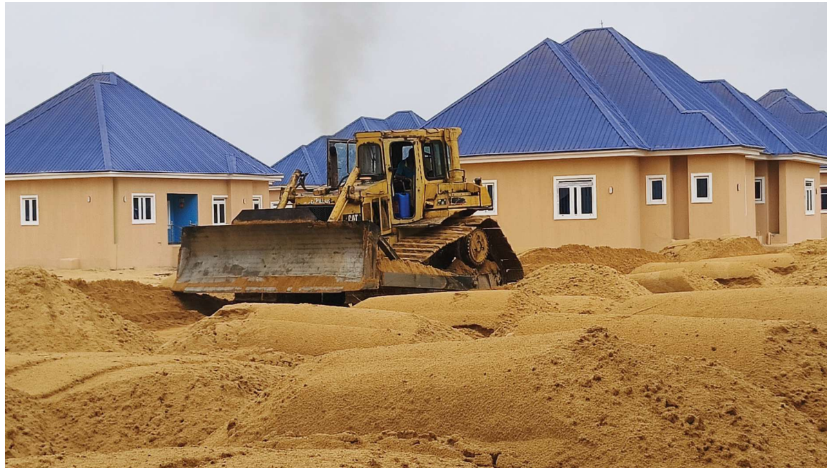
MOPOL BASE, SAMPOU ONGOING
