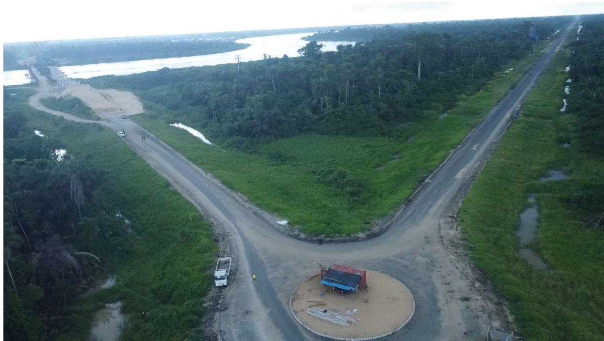
SHOWING THE ROAD TO OPOROMA ON THE RIGHT AND THE BRIDGE ON THE LEFT
