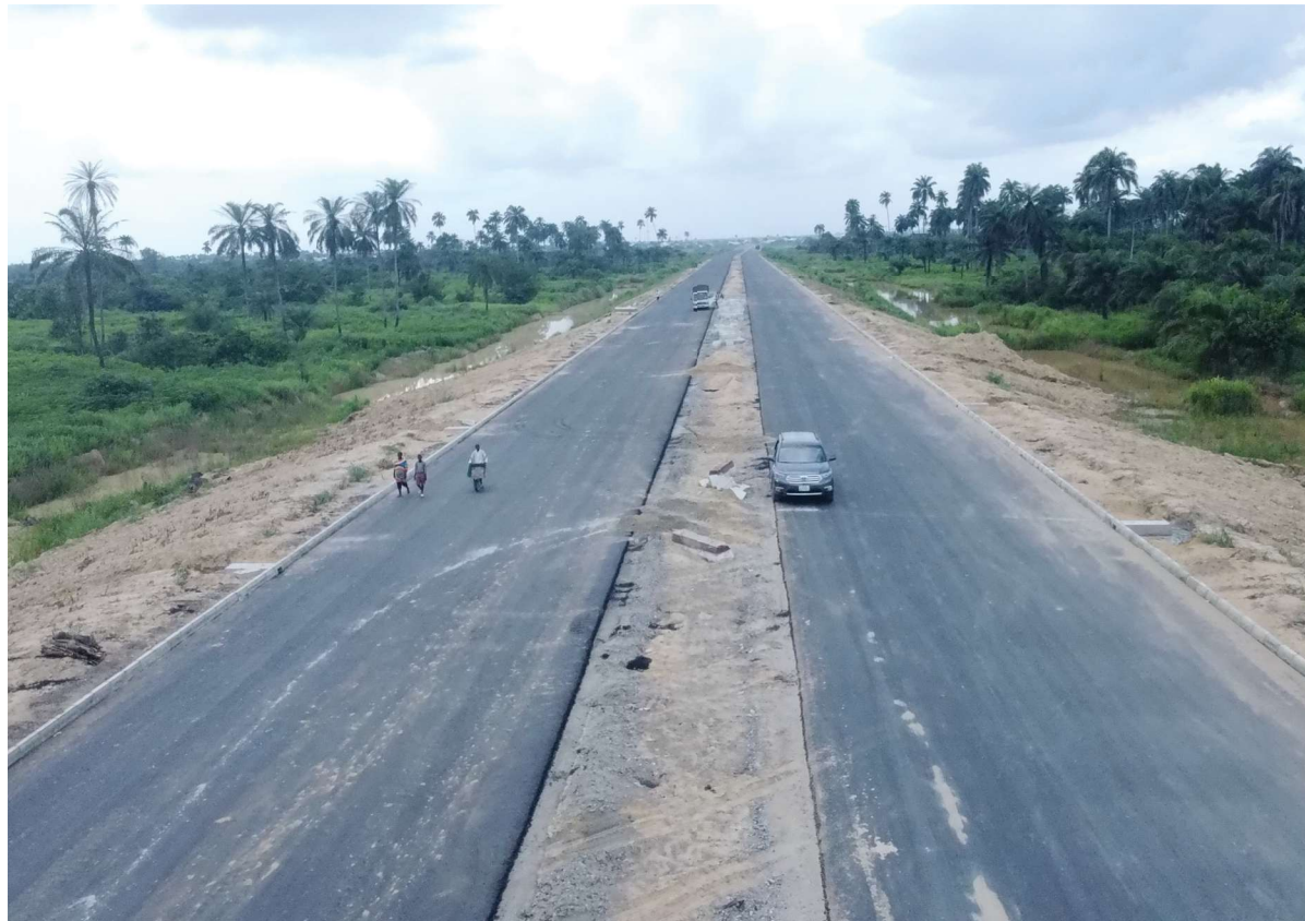
GLORY DRIVE PHASE 3, ABOUT 3KMs ASPHALTED
